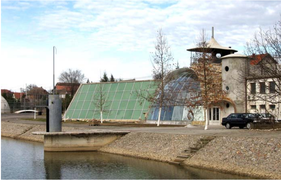
Figure 6 - Solar house with shell entirely made out of ferrocement (courtesy M. Milinkovic, Belgrade, Serbia).
