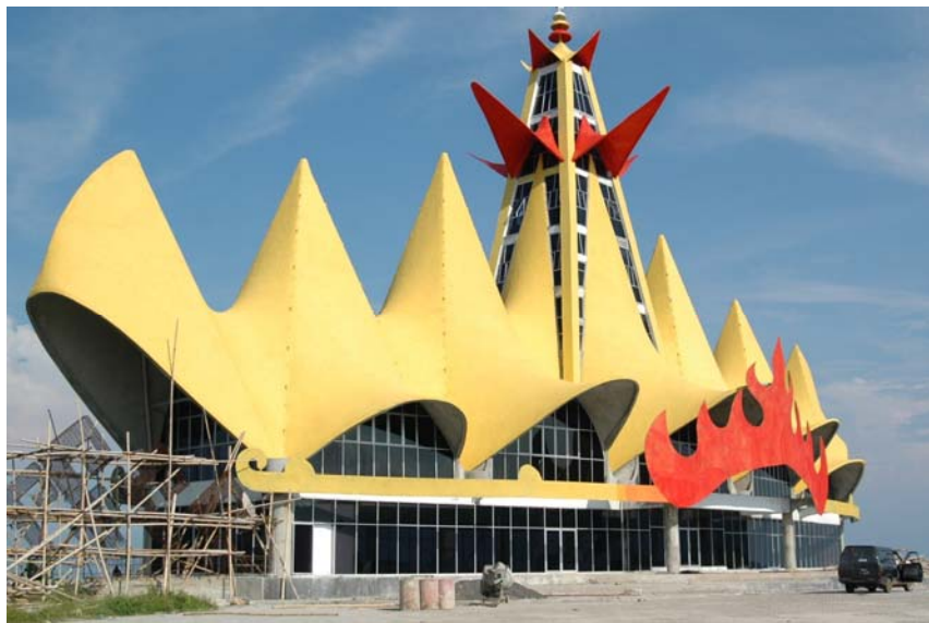
Figure 4 - Ferrocement roof of the Siger Landmark, South Lampung, Indonesia (courtesy A. Djausal and Bayzoni, Lampung, Indonesia).
