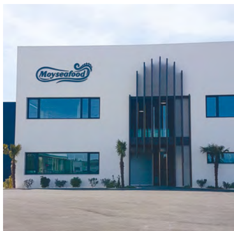
Industrial building enclosing, Cádiz, Spain
